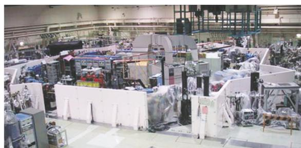
Fig. 2 Radiation shielding wall newly constructed for the top-up operation. The 53 m storage ring was completely surrounded by a lead wall 10 cm thick.
