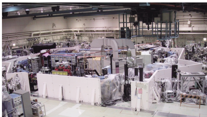
Fig. 7 (Color online) Reinforcement of the radiation shielding wall preparing for top-up injection.
