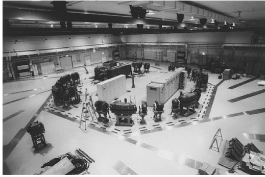
Fig. 3 UVSOR storage ring under construction.
